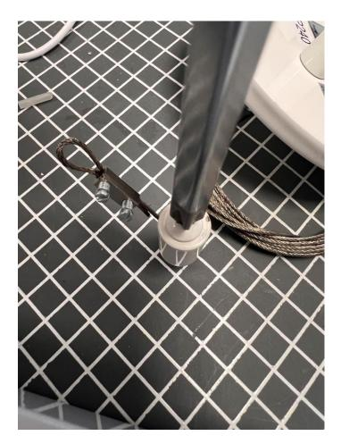
Remove the screw from the plunger with a Phillips head screwdriver
